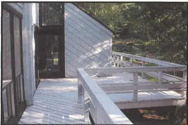
Northwest Elevation - Kitchen
