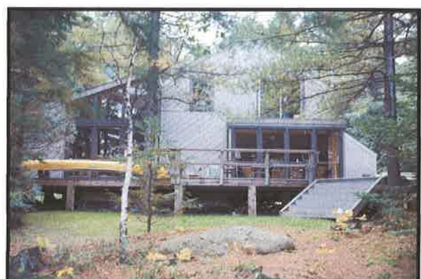
During Remodeling 1976 (Some railings not completed)
